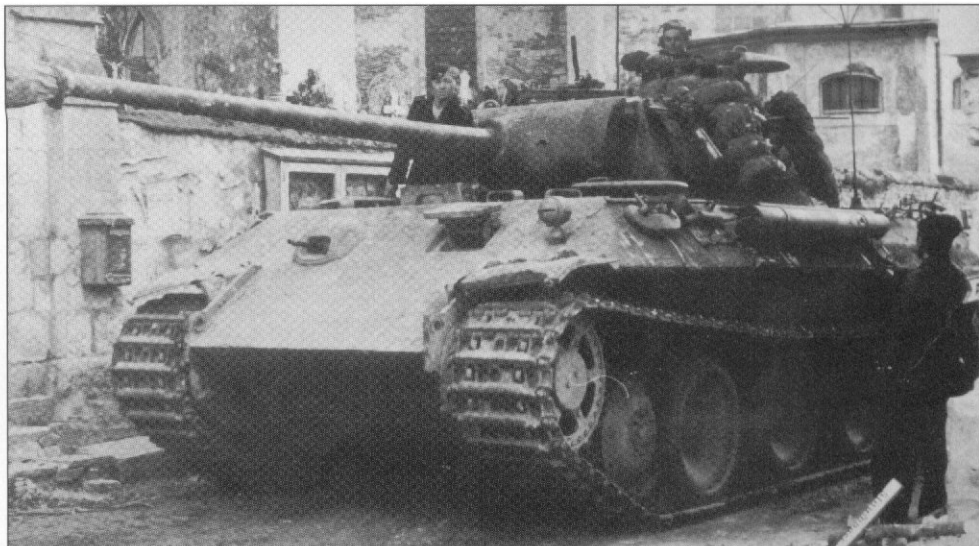
Another Pzbfswg Panther Ausf. A in a French town. Used as an Sd.Kfz. 267 (standard command vehicle for an armored unit) as well, it features the 6-foot (2 m) rod antenna fitted on the turret's roof, but the long-range star antenna is attached to the standard mount behind the turret. A possible reason for this unusual combination could be that the actual antenna mount was damaged. (F. Schulz)
