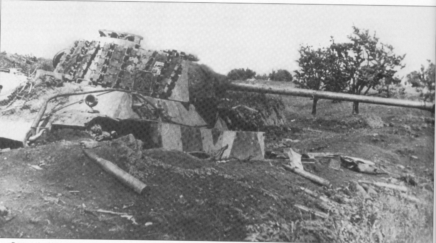
Destroyed at Vyskov, Czechoslovakia, another Ausf. G sits abandoned. The gun mantlet is of the late chin type. A lot of extra track links are stored on the turret. Its vehicle number, "215", is painted directly onto the track links. The camouflage scheme, diagonal green and brown stripes, was applied using stencils. (S. Netrebenko)
