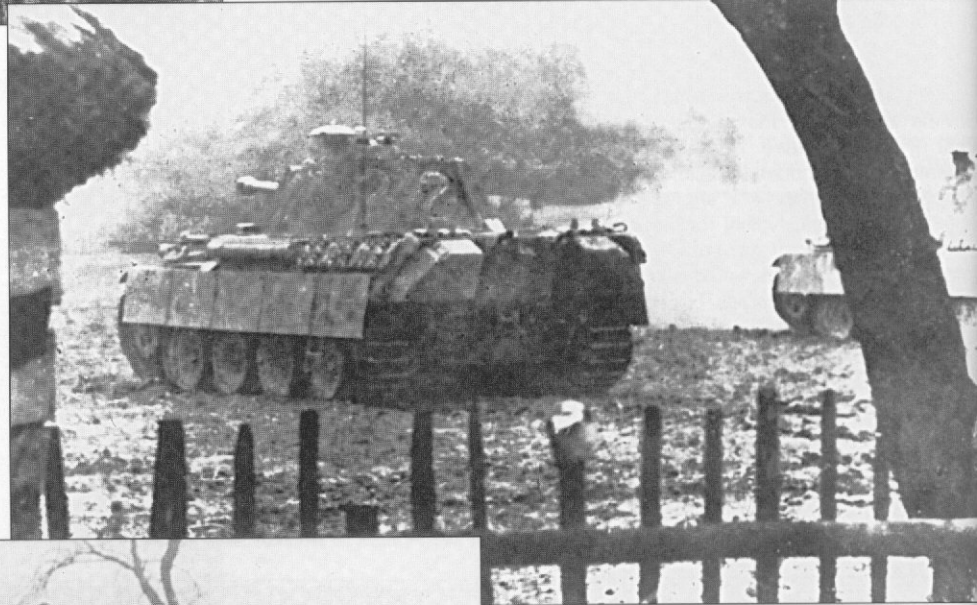
The crew of this Panther poses for a photo. This is an early Ausf. G, as the Zimmerit coating shows. The MG ball mount is shut up with a plug plate. (P. Kammann)
