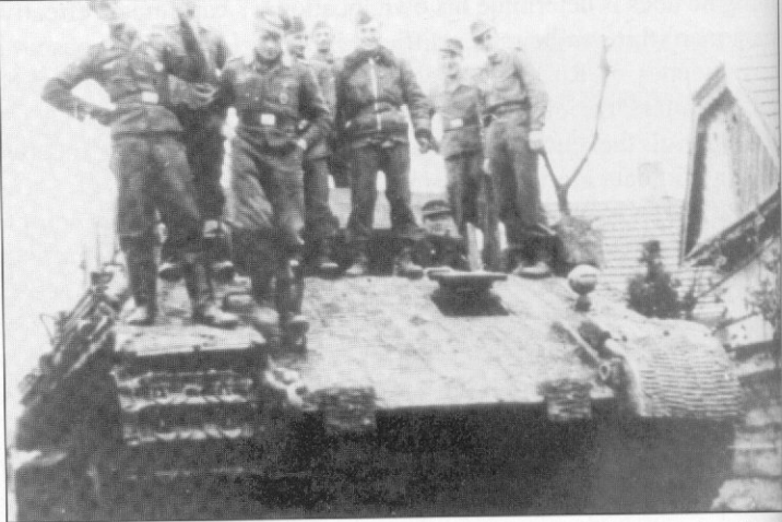
Lacking planes, these Luftwaffe troops pose atop a Bergepanther Ausf. D. This versatile recovery vehicle was probably the most important conversion of the Panther. The square steel plates attached to the bow are clearly shown. The crane is dismounted and stored on the right side of the hull. This Panther has received a complete coating of Zimmerit . (H. Hoppe)
