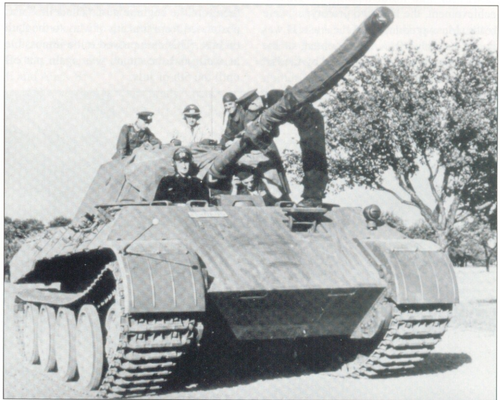
The Panther appeared in early 1943, and this photo gives a good impression of its shape. This vehicle shows a late Ausf. D, as evidenced by the fact that the right headlamp was deleted. The muzzle brake is not yet fitted, but the gun does show a protective cover. The Panther lacks all equipment, indicating that it is brand new. The unusual license plate shows a Berlin number (1A). Since the color of the vehicle appears to be dark grey, this well known photo has often been dated from 1942. (M.Green)
