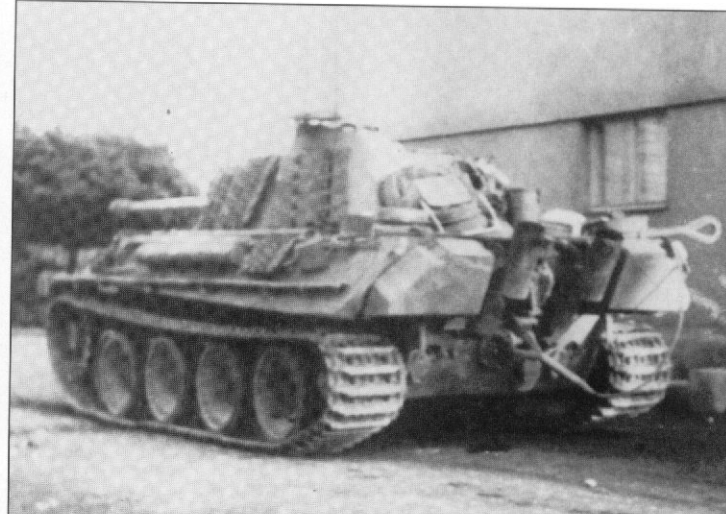
This undamaged Panther was abandoned at Tisnov, Czechoslovakia, at the end of April 1945. This is a very late Ausf. G fitted with a flame suppressor exhaust. A lot of extra equipment is carried on the engine deck and the turret. (S. Netrebenko)
