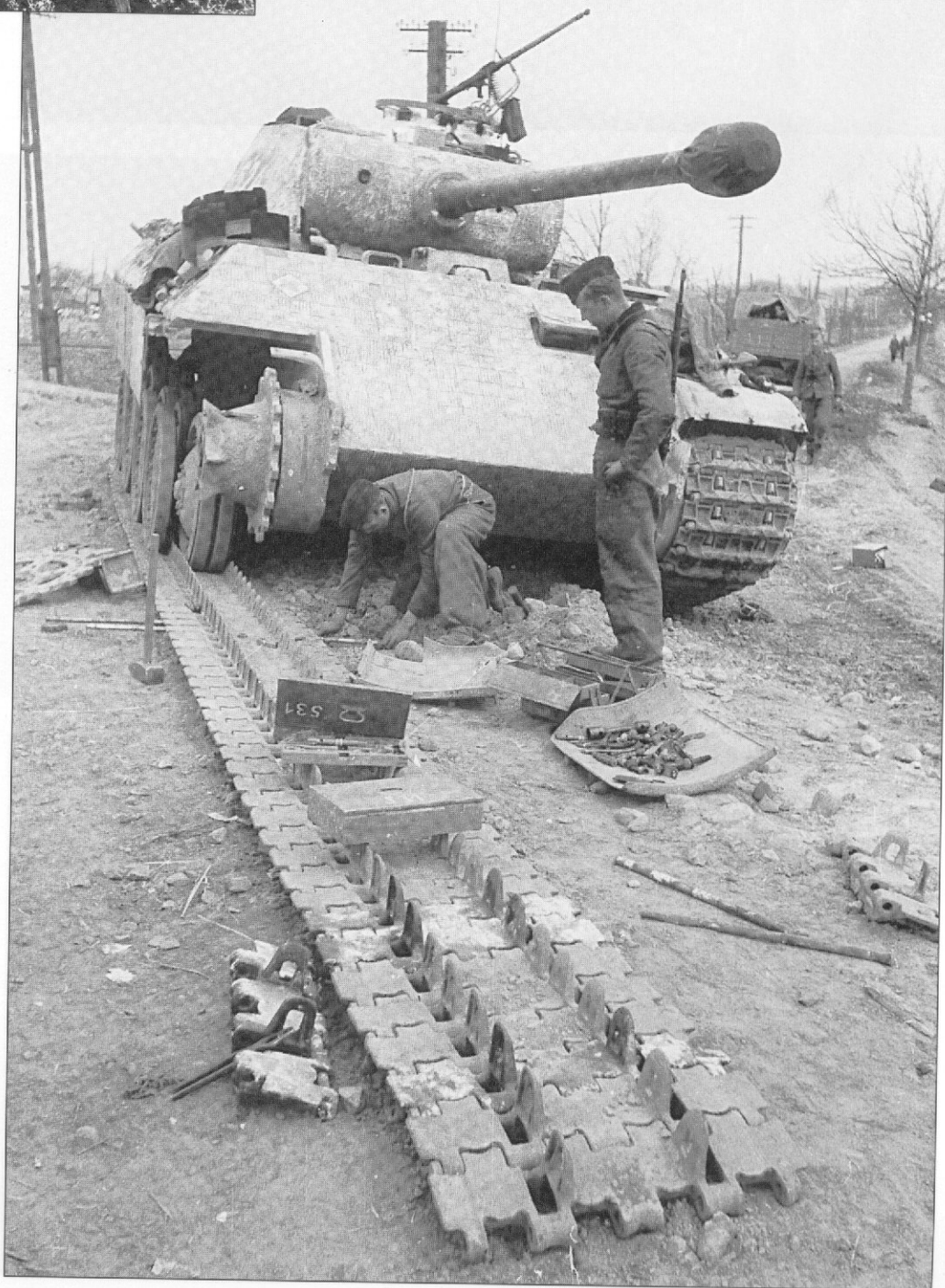
Panther number "633", an early Ausf. D of Pz.Abt. 52, was destroyed during Operation "Zitadelle". Note the pistol port cover hanging at its chain, which was possibly blown out by an internal explosion. Also, the armor skirt supports are visible. This arrangement was quite prone to damage, and many Panthers lost their skirts during combat. The crews often fixed additional brackets for them. A Panther head insignia is barely visible in front of the turret number. (S. Netrebenko)
